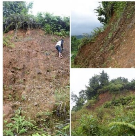
Figure 8. Landslides in Mangkutana Sub-District
